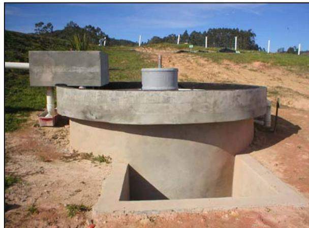
**Figura 15.** Reator UASB
