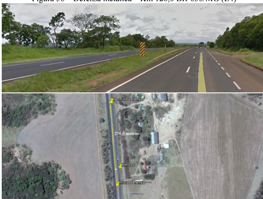
Figura 56 – Defesa metálica – Km 126,0 BR-050/MG (L4)
