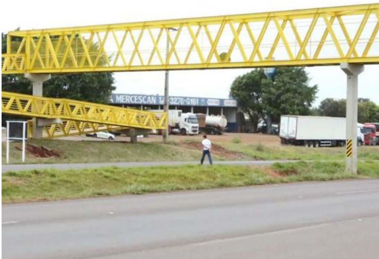
Figura 26 – Travessia irregular de pedestres – Rodovia BR-467 (Toledo - PR)
