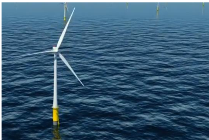
Figura 21 – London Array Offshore Wind Farm .
