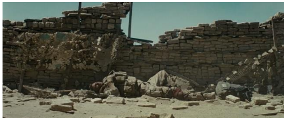
Fig. 126. The partially destroyed wall
