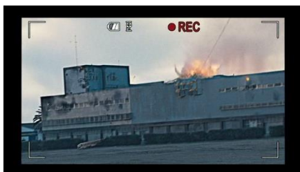
Fig. 85. The material destruction in Nasiriyah
