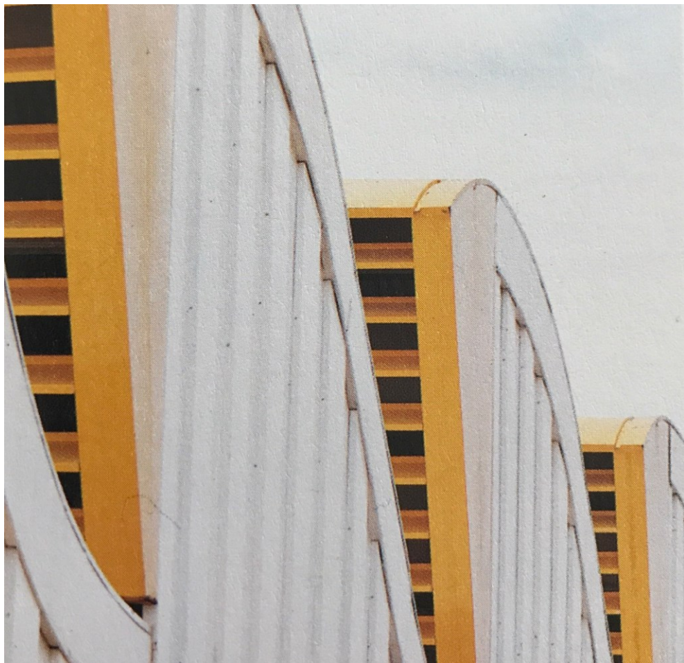
Figura 54: Sheds do CRTS
