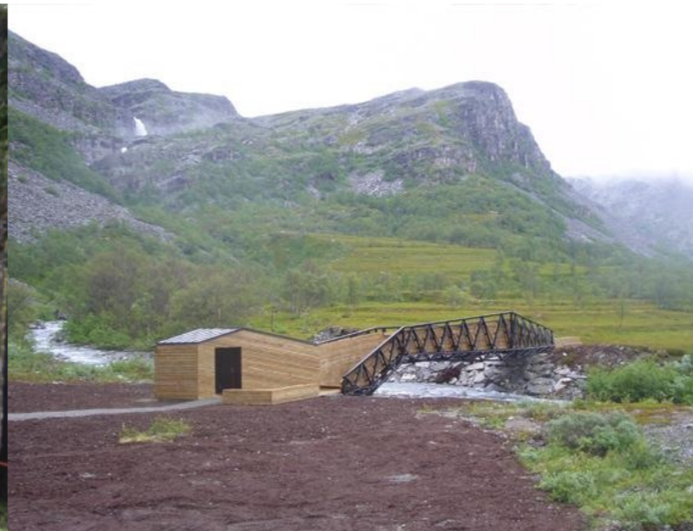
Lillefjord Rest Stop. Pushak Architects
