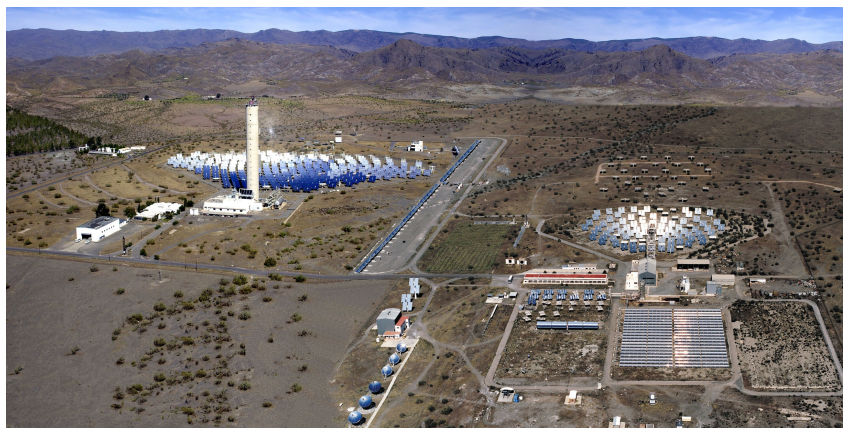
(a) Facilities and laboratories available at the Plataforma Solar de Almería.
