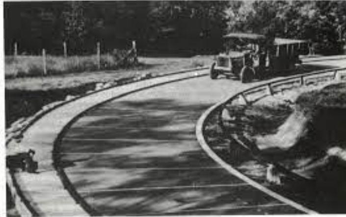
Figura 2.2 - Bureau of Public Roads test track.
