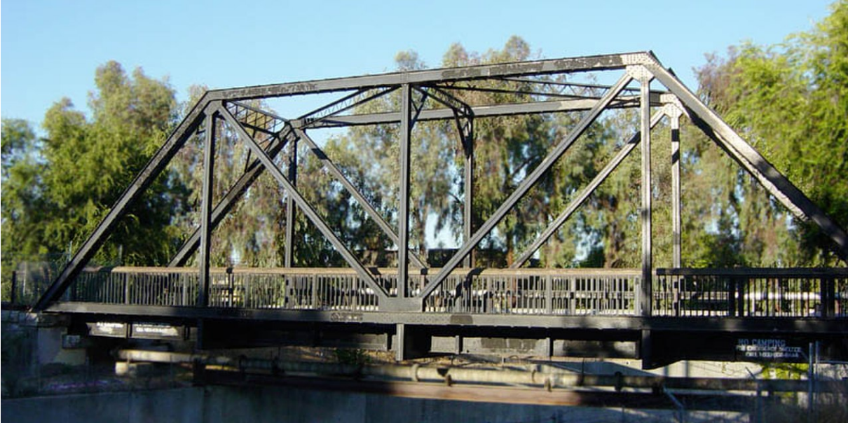
Figura 18 – Ponte Southern Pacific Railroad.
