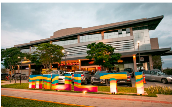
Figura 12 – Fachada do Multi Open Shopping
