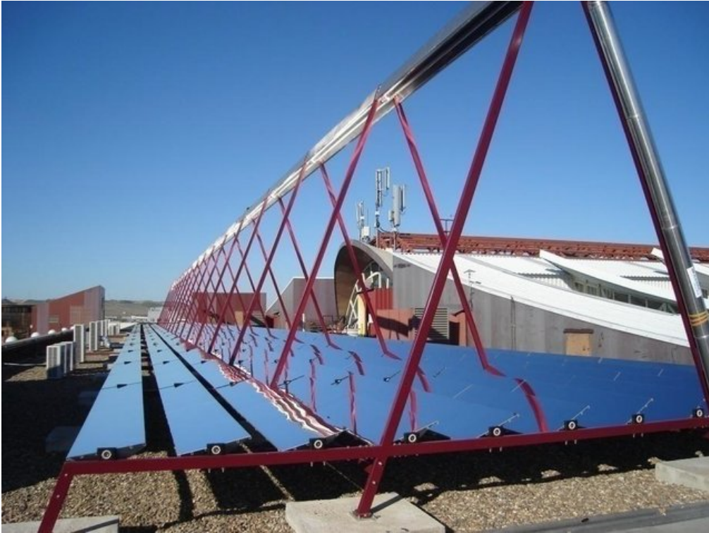
Figure 1: Fresnel solar collector installed at ETSI absorption solar plant [23].
