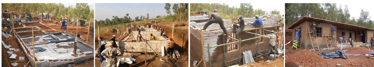
Figura 3: MASORO VILLAGE PROJECT. Archdaily, 2013. Disponível em: [https://www.archdaily.com.br/br/01-153361/masoro-village-project-slash-ga-collaborative] . Acesso em: 23/01/2024.
