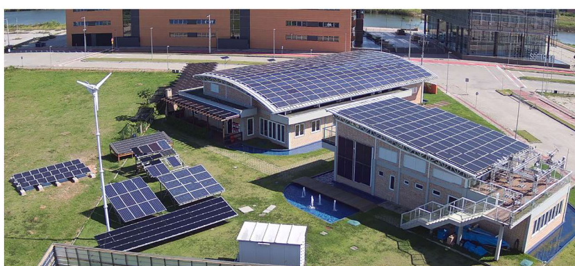
FIGURE 4 Aerial image of the three PV systems analyzed in this study and the objects nearby that cause shading on the systems during certain times of the day and year [Colour figure can be viewed at wileyonlinelibrary.com ]
