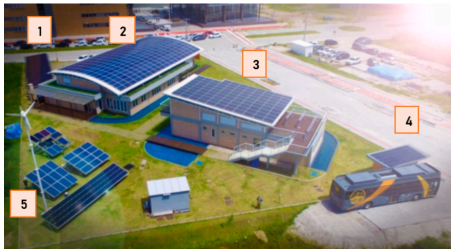
Fig. 2. Aerial view of the Solar Energy Research Laboratory at Universidade Federal de Santa Catarina in Florianópolis-Brazil with the e-Bus, which represents the largest single load during battery charging for 1-hour periods five times/day shown at the bottom right.
