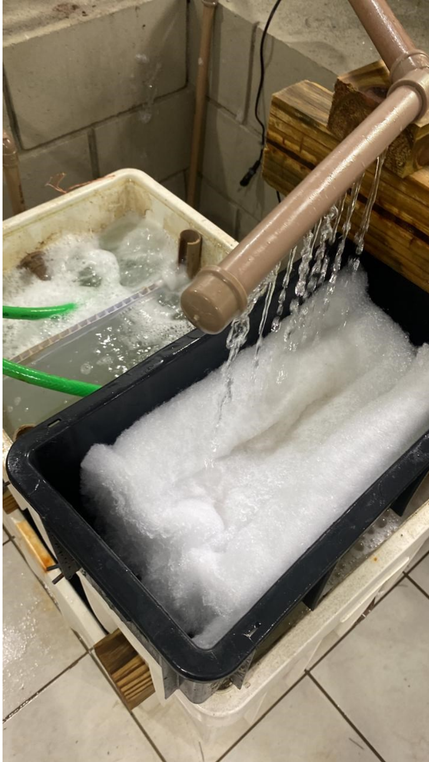
Apêndice D - Mechanical filter filled with polyester fiber to retain suspended solids. Photo by Marcelo Santana
