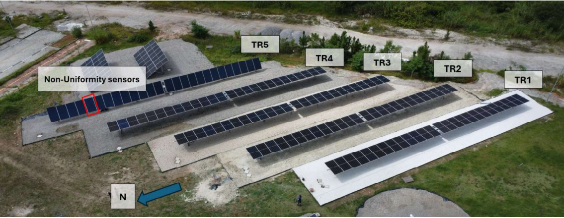
Fig. 1. Research PV pilot plant composed of six distinct PV systems with varying albedo conditions. Systems analyzed include TR1 (white gravel), TR2 (kaolin), TR3 (sand) and T4 and TR5 (gray gravel).
