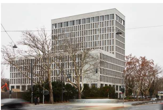
Figure 105. DIPF. Photo: Oliver Rieger. Source k9architekten.
