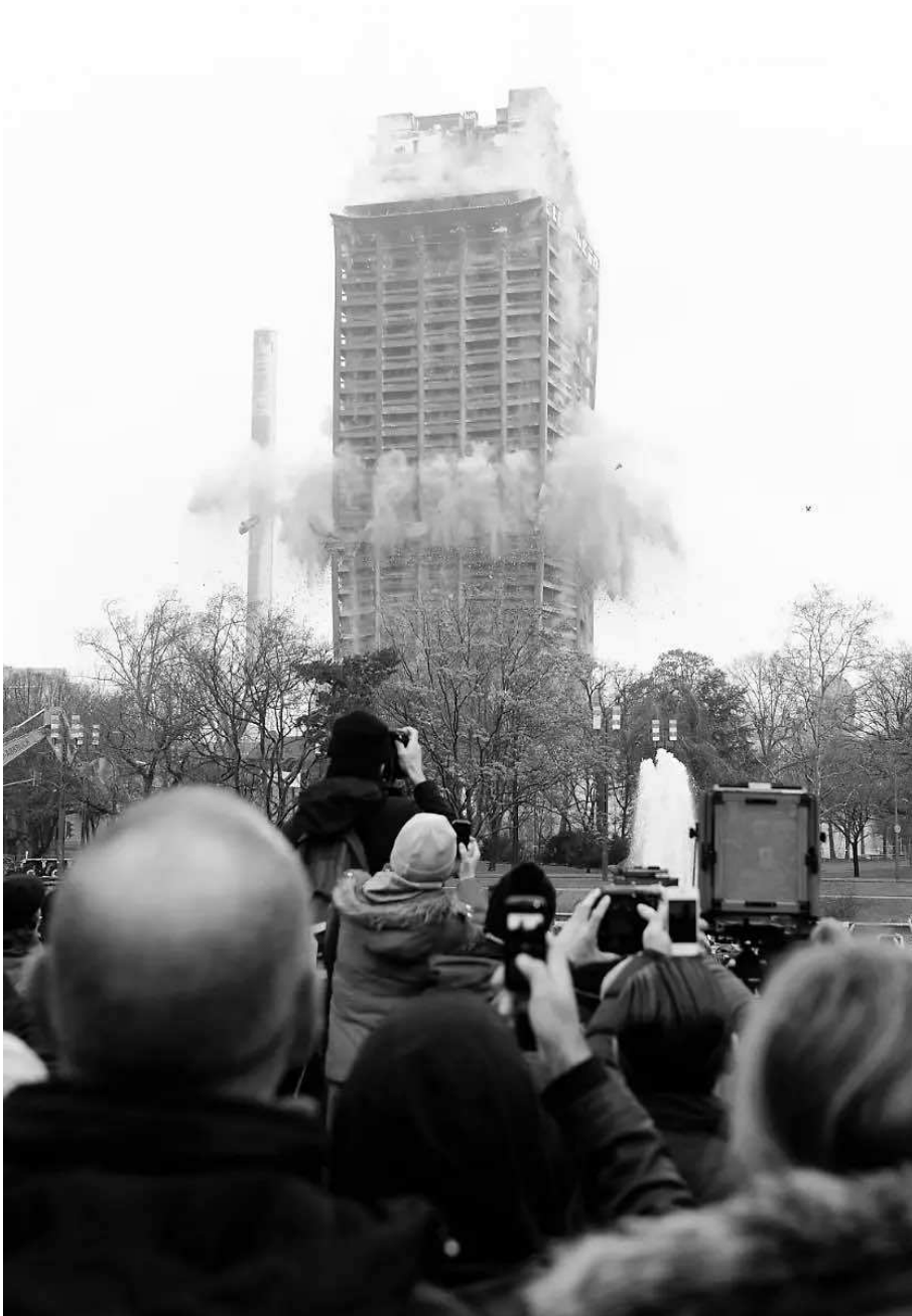
Figure 27. On February 2, 2014, people watch and photograph the demolition of the AfE tower. Source: Deutsche Presse-Agentur.
