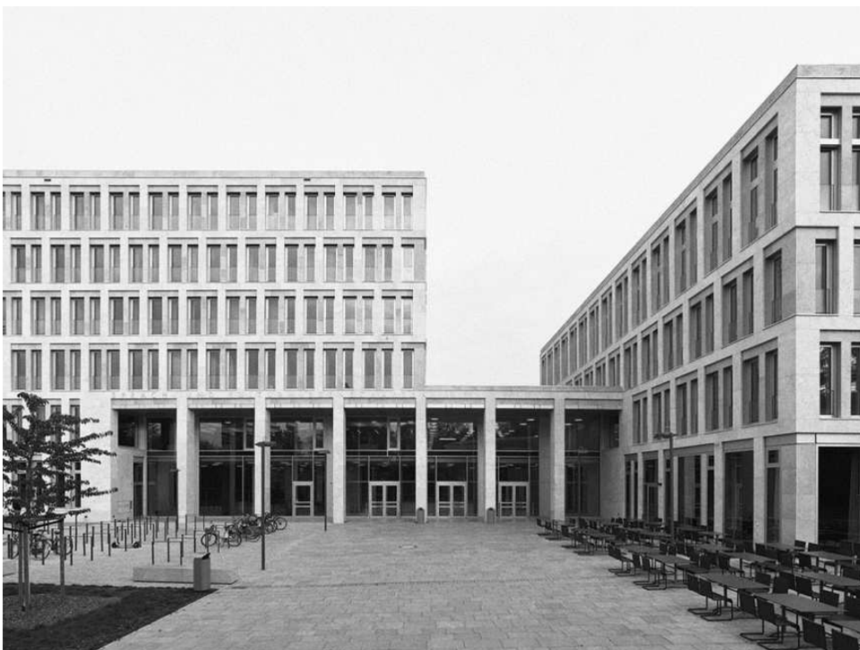
Figure 100. SKW's main entrance. Source: BLK2 Architekten.
