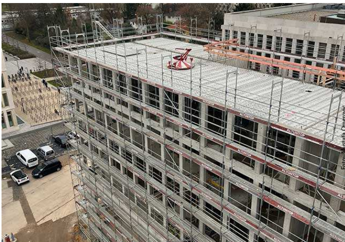
Figure 107. CFH under construction; May 2025. Photo: Mustafa Omrovic.
