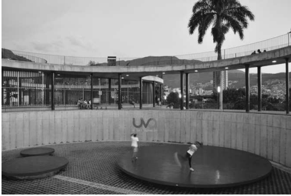
Figure 128. UVA de la imaginación, San Miguel. Here, the existing water infrastructure has been repurposed to create a multi-functional community centre. As shown, the tanks were opened to accommodate a programme that ranges from open-air theatres and walking trails to exhibition spaces and specialist music rooms. 2018.
