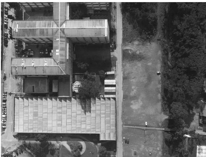
Figure 138. View of the HU as built. The expansive car park on the right borders the hospital, establishing a complex relationship with the watercourse traversing the campus. 2019. Photo: Felipe Finger. Source: LEUr UFSC.
