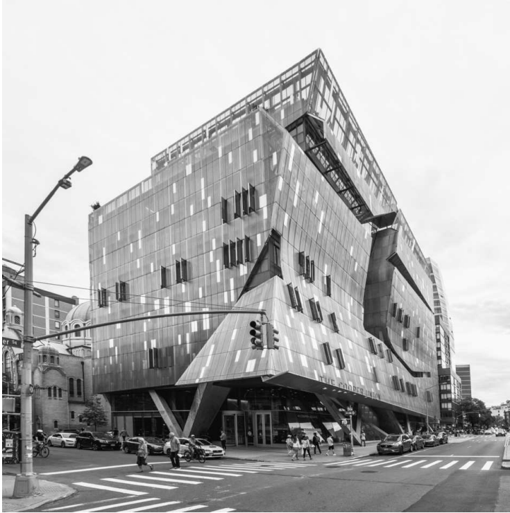
Figure 70. Cooper Union's Albert Nerken School of Engineering. Designed by Thom Mayne, Morphosis + Gruzen Samton-IBI Group. Photo: Ajay Suresh, 2019. Source: WM Commons.
