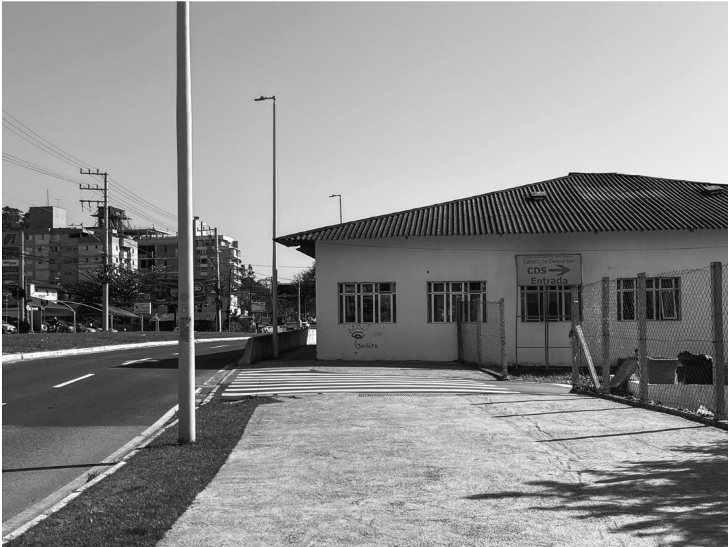
Figure 139. The building, which the city government had pledged to, now partially occupies the pavement. Its occupants must contend with the incessant traffic noise. 2024.
