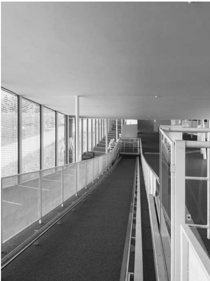
Figure 58. Accessibility platform inside the RLC. 2024.
