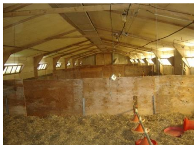
Fig 5 – Inside shed aspect
